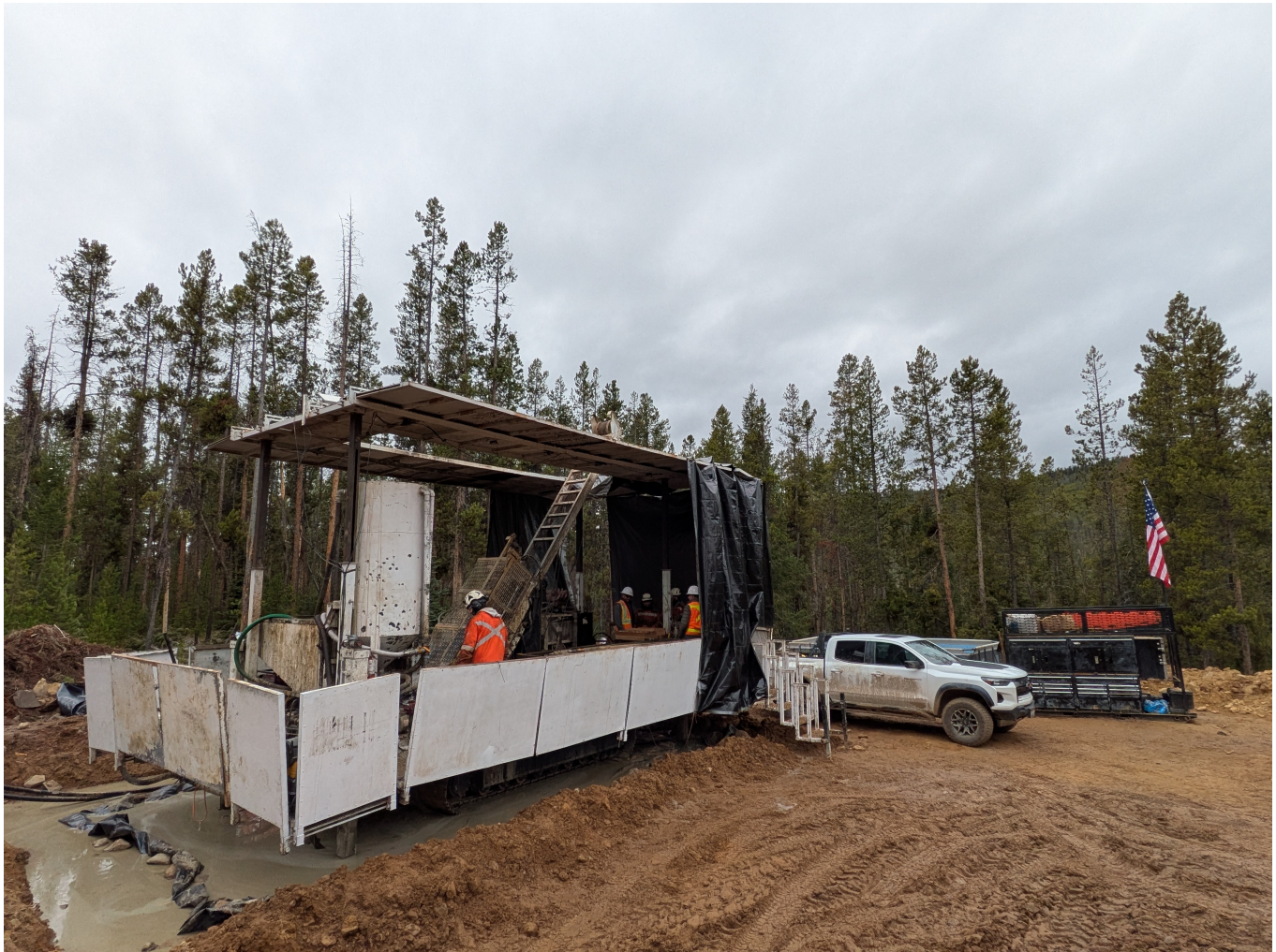
A drill rig at Joss at Beartrack-Arnett in Idaho, USA | Credits: Paul Harris
